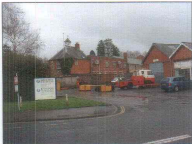
Site access from East Street
