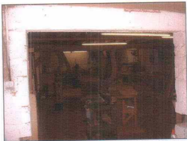
Internal photos showing restricted headroom and work space
