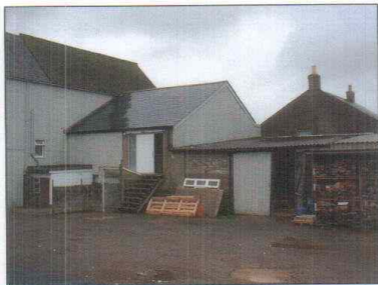
Ground level store and first floor workshop access.
